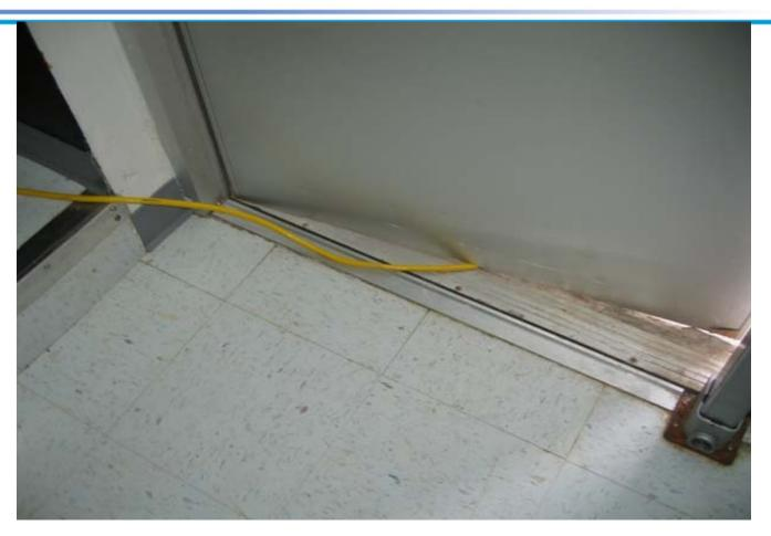
Electrical wire and flexible cord passing through work areas shall be protected from damage (including that caused by foot traffic, vehicles, sharp corners, protections, and pinching).
